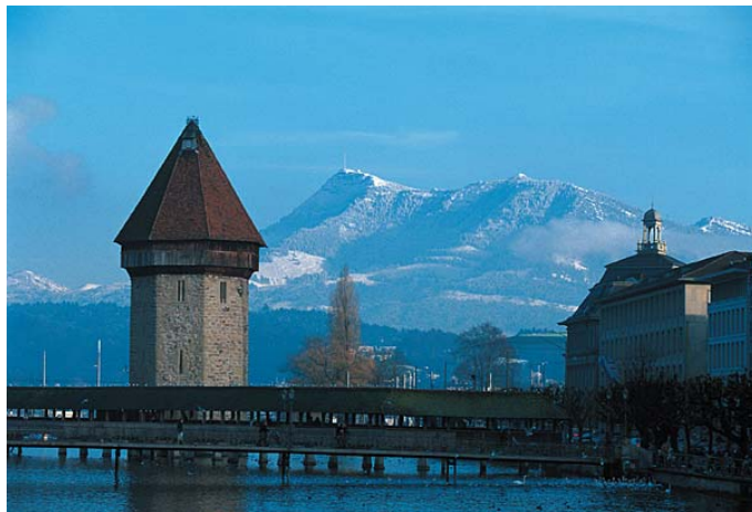
The famous Chapel Bridge in Lucerne, the oldest wooden bridge in Europe
